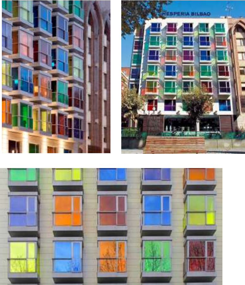
Fig. (6) Colored Glass façade’s windows of Hotel Hesperia, Bilbao, Bizkaia, Spain, 2005
