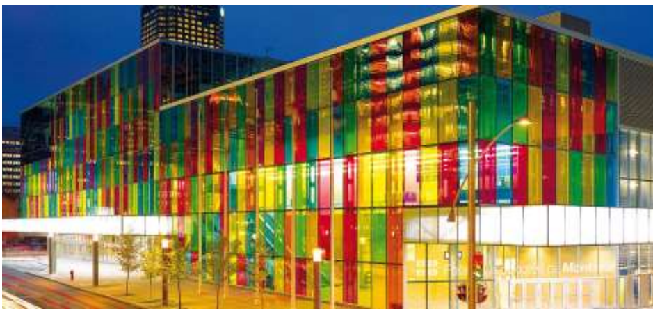
Fig. (7) Colored Glass façade at the Palais des Congrès, Montreal, Canada, 1999
