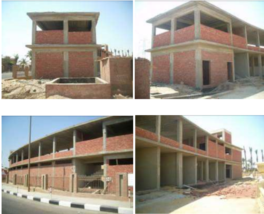
Fig. (9) showing the building to be beautified
